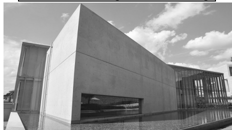
South Building (South Wing)
